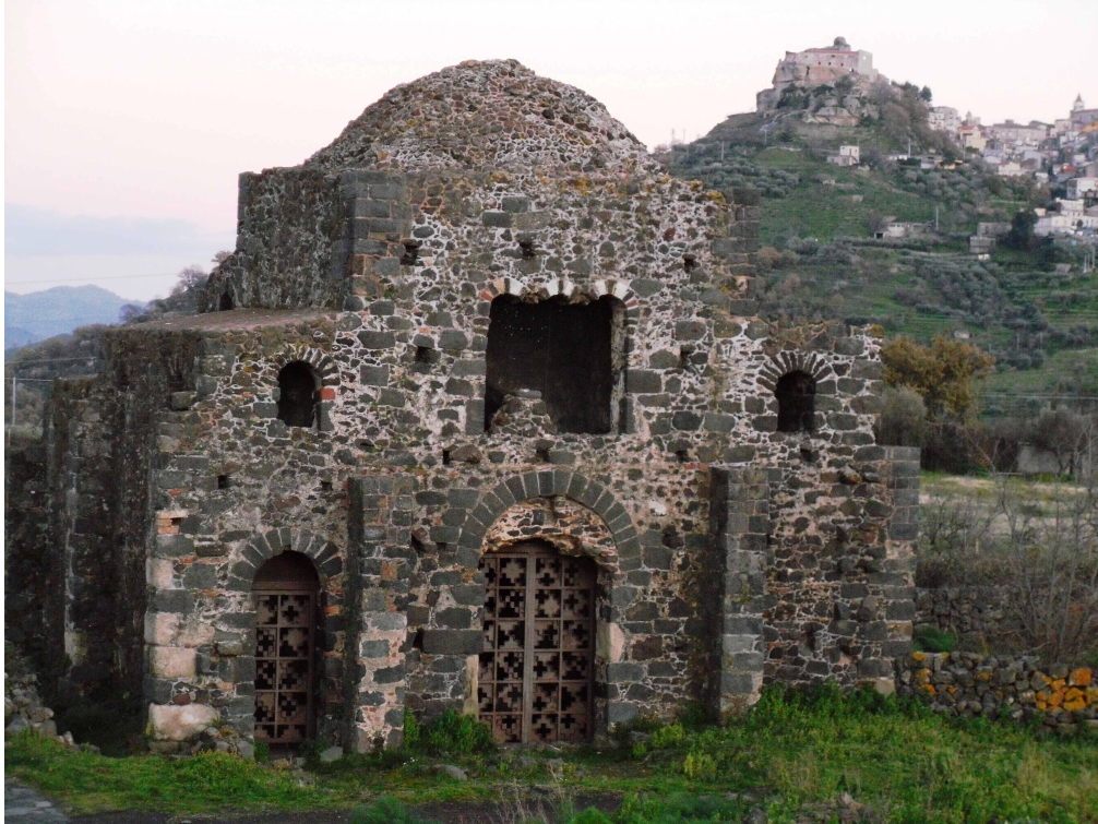
Main facade of the Cuba (Fondo Ambiente Italiano)
